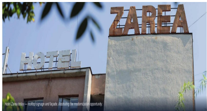
Current condition — rooftop signage & façade.
